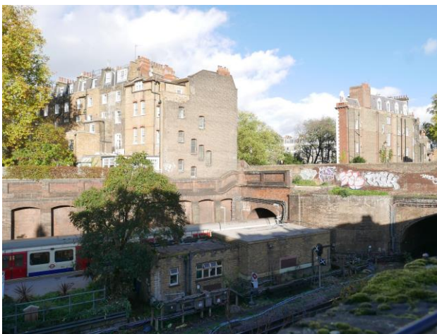
The sub-surface station looking towards the extended ticket-office, the glazed roof of the Edwardian booking-hall and the red-brick administrative building above the eastern-side of the Station Arcade; the surviving, early-20 th platform-canopies and the original, northern, arcaded revetment of 1868, with the rear elevations and trees in the gardens of the listed terrace at nos. 2 to 18 (even), Thurloe Street beyond; and the open area between the east of the station platforms and the bridge carrying the road from Pelham Street to Thurloe Square, with the original, plain brick, northern revetment of 1868 and the flanks of no. 52, and no 5, Thurloe Square, rising-up beyond.
