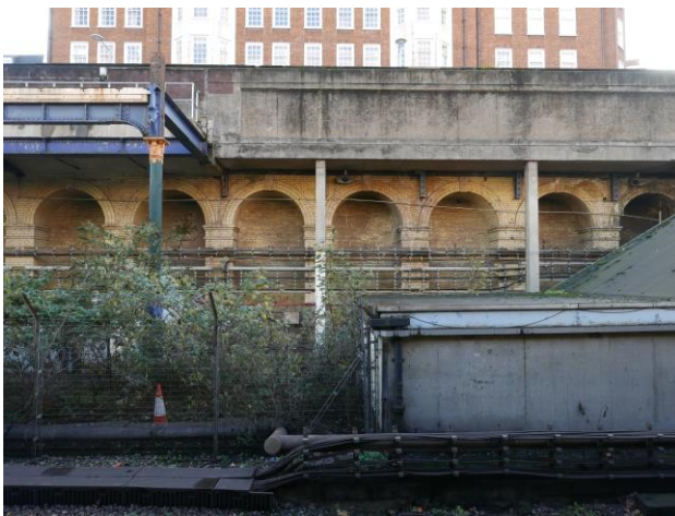
The later, 1870, arcaded southern revetment of the original sub-surface station with the modern brick and reinforced-concrete walls along the northern side of Pelham Street above, together with the surviving, free-standing, cast-iron columns that once supported the southern edge of the long-lost, elliptical-arched, glazed roof and sloping glazed roof above the Metropolitan District Railway's single-ended reversing-bay and the adjacent platform of the original sub-surface station
