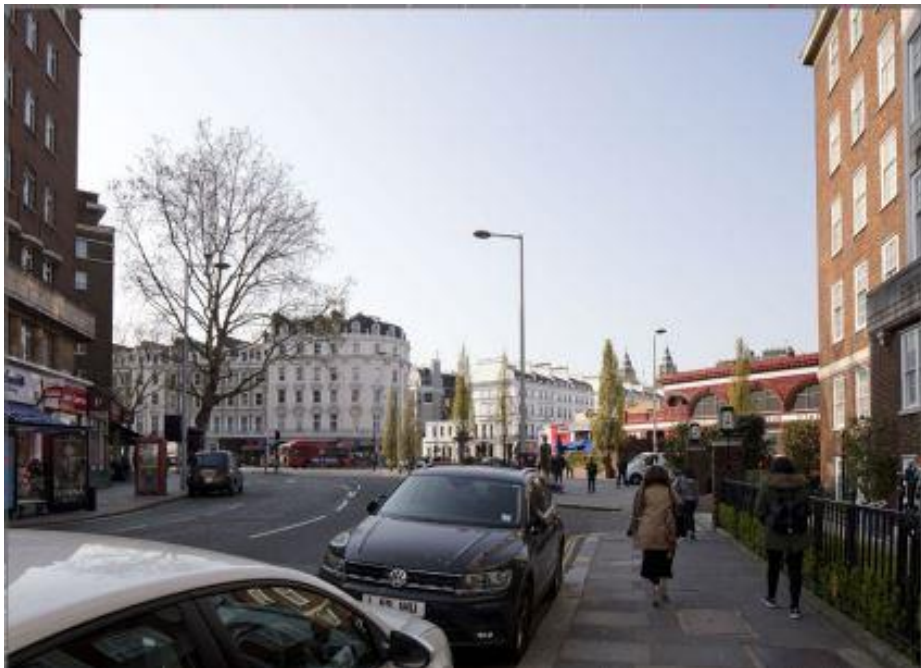
THE APPLICANTS' AS EXISTING AND AS PROPOSED VERIFIED VIEW 08 SHOWING THE PROPOSED DEVELOPMENT AROUND 'THE BULL-NOSE' CURVE AS SEEN FROM THE NORTH-EASTERN SIDE OF THE ROAD FROM ONSLOW SQUARE LOOKING NORTH-WESTWARDS
