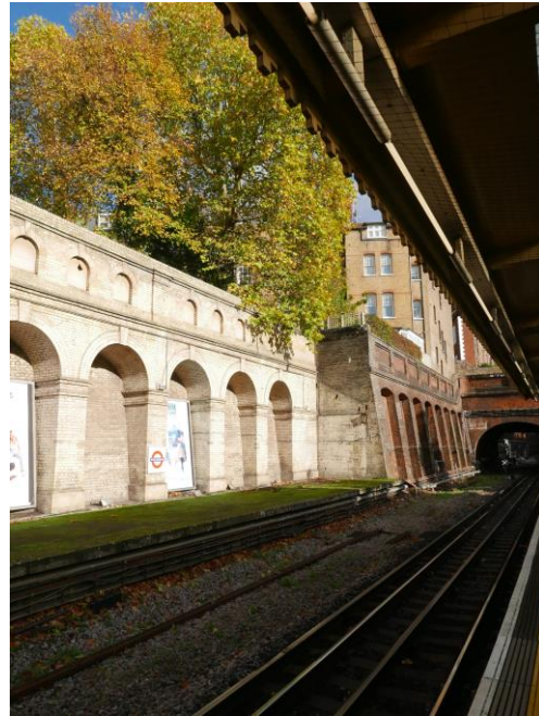
The western and eastern ends of the original, arcaded revetment of 1868 along the long disused northernmost platform of the sub-surface station, with the rear of nos. 20 to 34, Thurloe Street, and the trees in the gardens in the gardens of the listed terrace at nos. 2 to 18 (even), Thurloe Street rising-up above the wall
