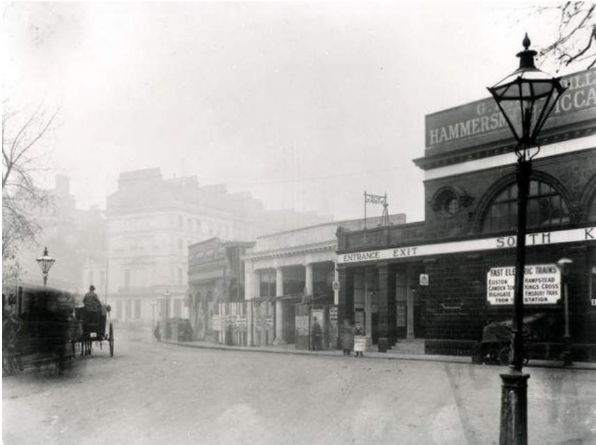
The new entrance to the Metropolitan Railway and Metropolitan District Railway station and Station Arcade from Pelham Street nearing completion, showing the remains of earlier buildings to the LH side and Leslie Green's surface-level station building for the UERL's Great Northern, Piccadilly and Brompton Railway to the RH side
