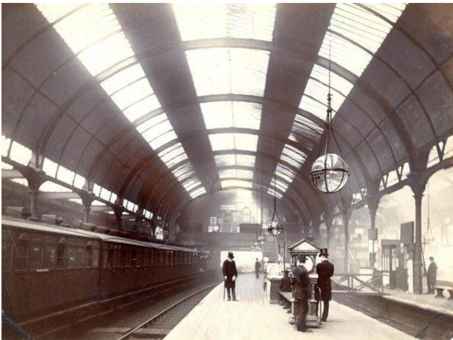
The interior of the central part of the sub-surface station looking westwards showing the elliptical-arched, glazed roof above the Metropolitan District Railway westbound and eastbound tracks on the LH side and the original Metropolitan Railway reversing-bay on the RH side, and the island platforms to each side
