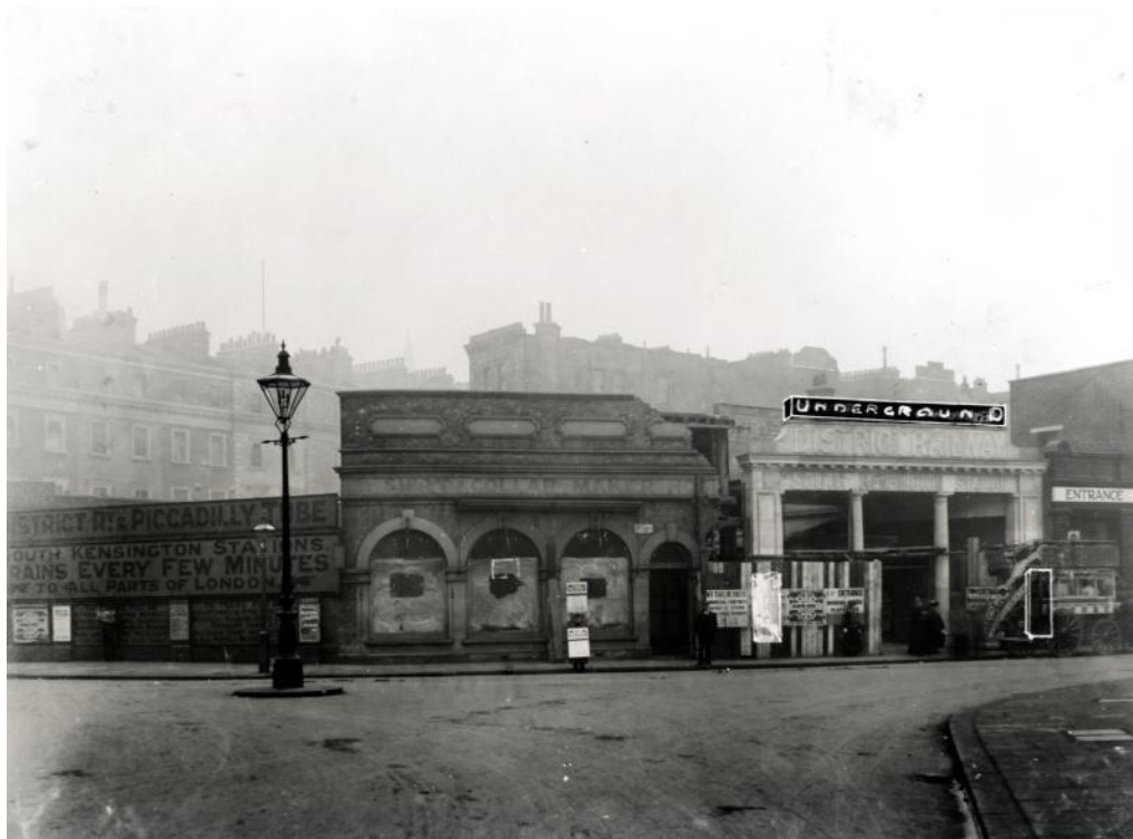
The new entrance to the Metropolitan Railway and Metropolitan District Railway station and Station Arcade from Pelham Street nearing completion, showing the remains of earlier buildings and the low-wall and hoarding around the ventilation opening above the tracks to the west of the station to the LH side and the entrance-wing to Leslie Green's surface-level station building for the UERL's Great Northern, Piccadilly and Brompton Railway to the RH side
