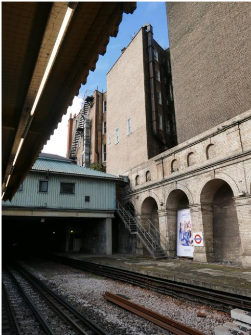
The western and eastern ends of the original, arcaded revetment of 1868 along the long disused northernmost platform of the sub-surface station, with the rear of nos. 20 to 34, Thurloe Street, and the trees in the gardens in the gardens of the listed terrace at nos. 2 to 18 (even), Thurloe Street rising-up above the wall
