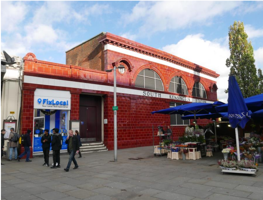
Leslie Green's surface-level station building for the UERL's Great Northern, Piccadilly and Brompton Railway fronting Pelham Street, showing the surviving original but unused single-storey entrance-wing on western (LH) side. The empty site of the original single-storey exit-wing on the eastern (RH) side - demolished in 1973-1974 - concealed by the tree and the florist's umbrellas
