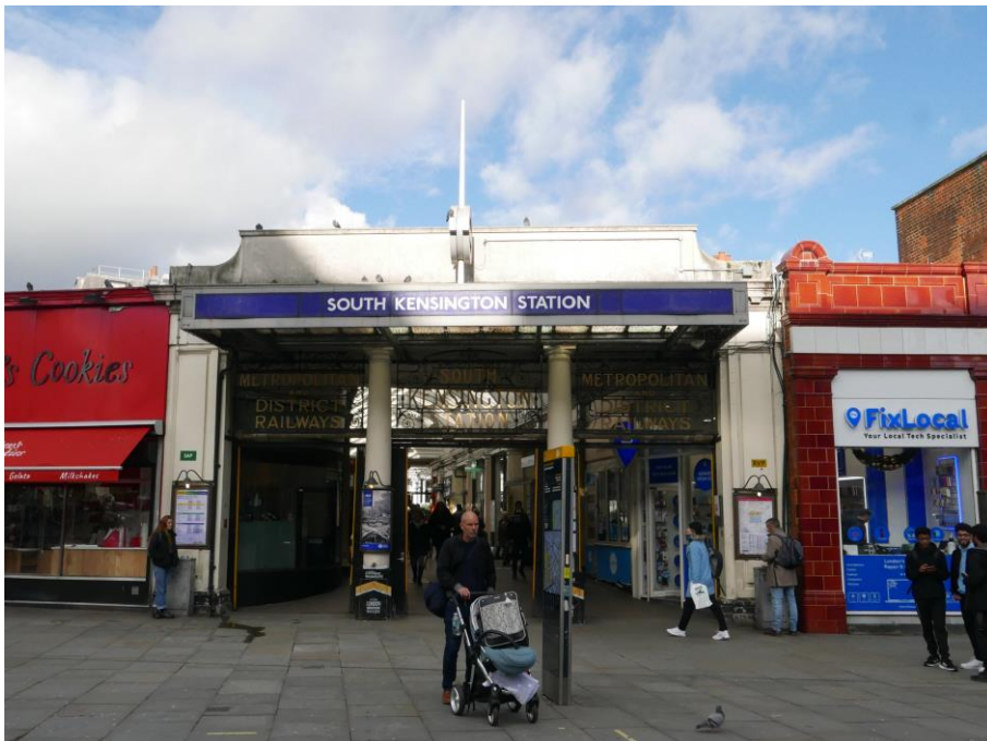
The Pelham Street entrance to the Station and the Station Arcade
