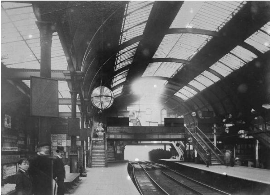
The interior of the southern side of the sub-surface station looking westwards showing the shallow pitched, glazed roof above the original Metropolitan District Railway reversing-bay on the LH side, the elliptical-arched, glazed roof above the Metropolitan District Railway westbound and eastbound tracks, and the island platforms to each side
