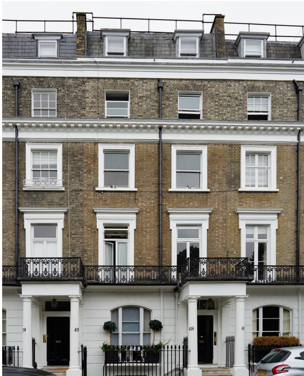
PHOTOGRAPGH SHOWING VERTICAL GRADUATION OF FENESTRATION AT 48-49 THURLOE SQUARE
