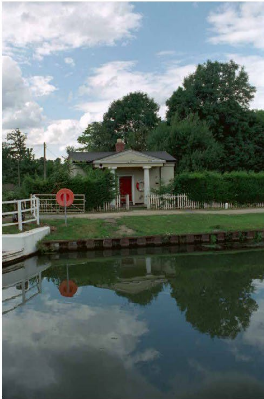
Figure 1 Bridgekeeper's House, Fretherne Bridge, Fretherne, Gloucestershire. One of a series of classically-inspired houses along the Gloucester-Sharpness canal of the early nineteenth century. Probably designed by Robert Mylne who had acted as Surveyor to the company in 1793. A high degree of architectural interest and individuality is given to what is more usually an unremarkable building type. Listed Grade II.
